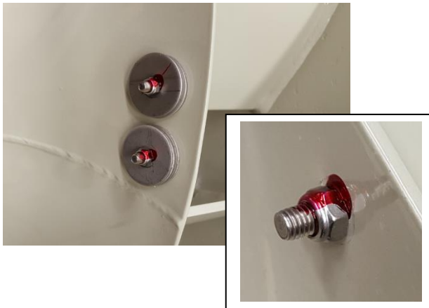
Figure: Bolt markings, visual inspection
